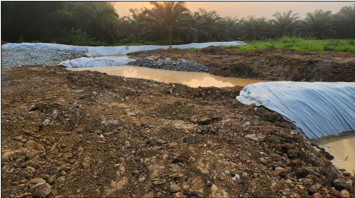
Figure 22 : Construction of silt trap at TSF2 Cell 3 area.
