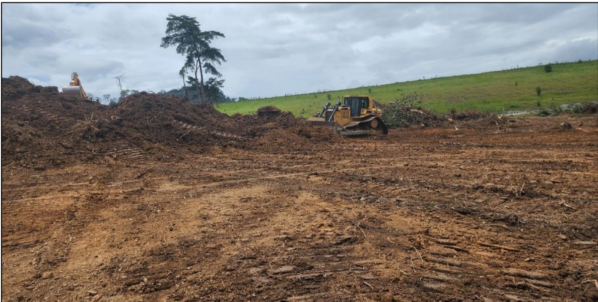
Figure 21 : Topsoil stripping and stockpiling.
