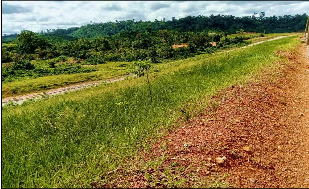
Figure 48: Outer slope stabilization with grass at TSF 2 Cell 2 main embankment
