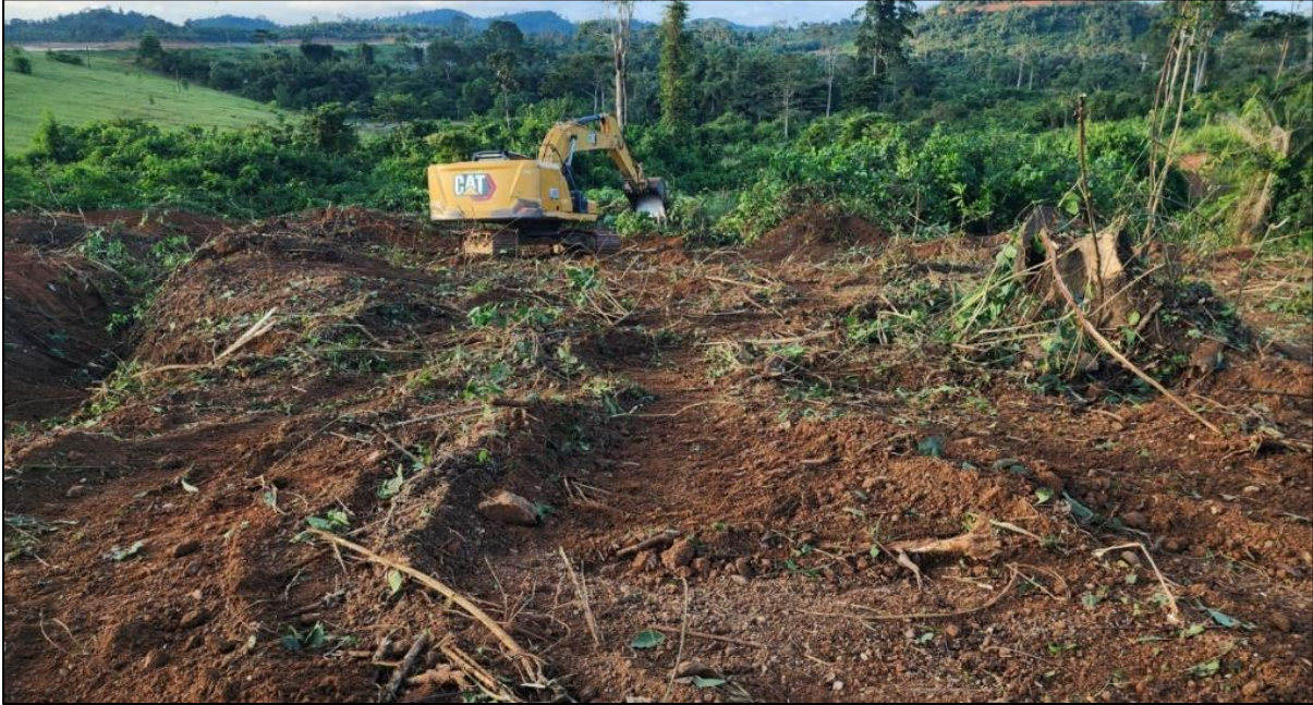
Figure 20 : Vegetation clearing at TSF 2 Cell 3..
